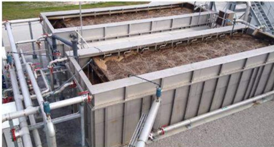
Note(s): Image represents secondary treatment which includes biological degradation of organics matter
