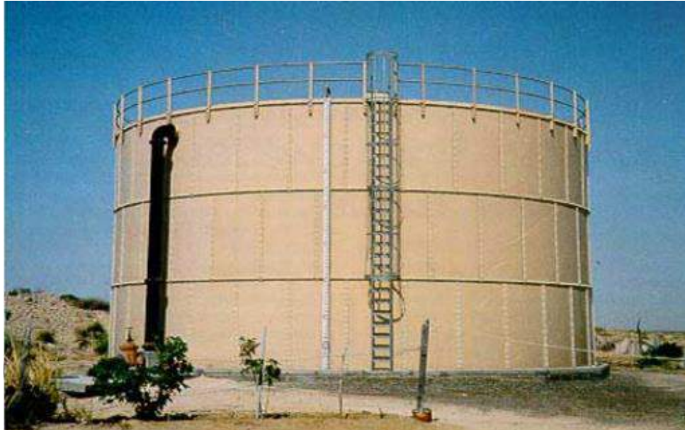
Note(s): Image represents storage of treated wastewater
