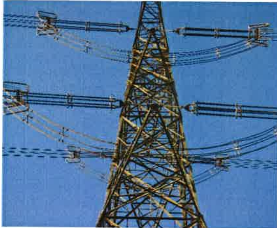
765 KV D/C Gadarwara STPS-Jabalpur Pool Line:
