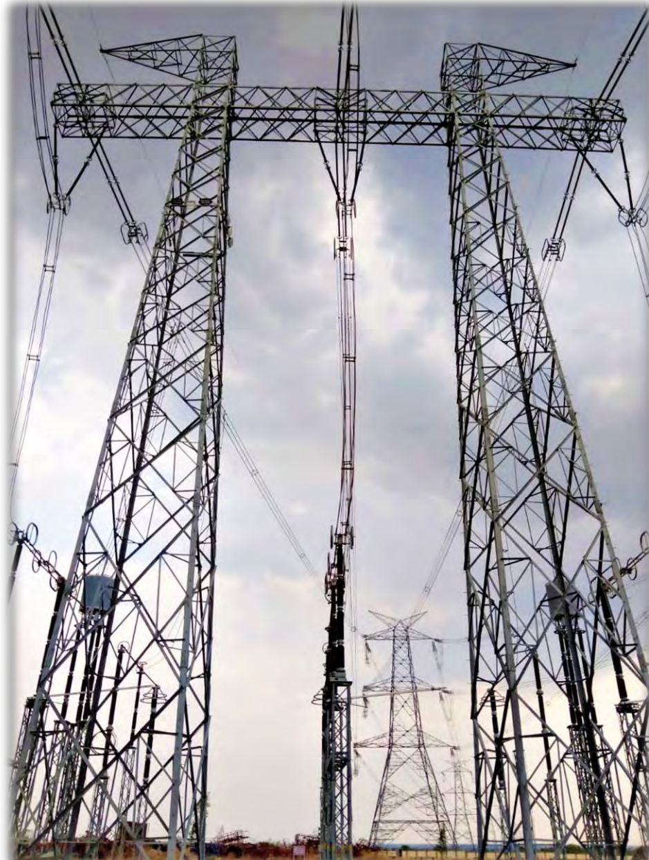
2x1500 MVA, 765/400kV Parli New S/S
