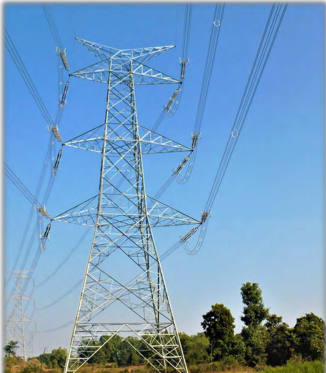
765 kV D/C Jabalpur - Vindhyachal Line
