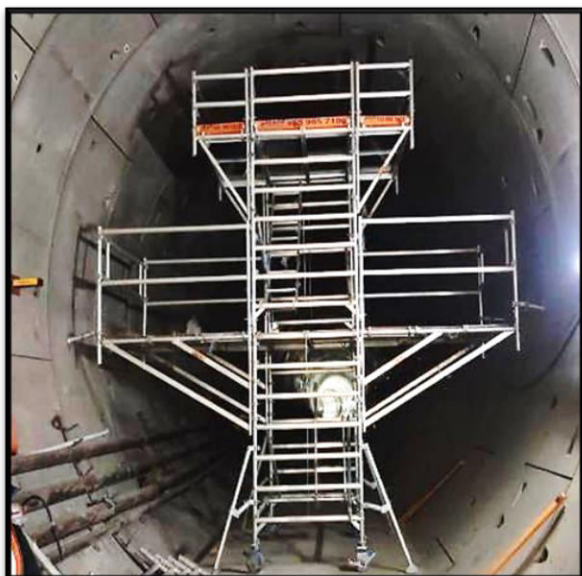
Supply of Aluminium Scaffolding (Model MWS054) for Chennai Metro Terminal Project, Tamil Nadu
