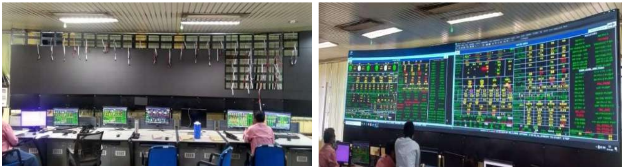
Active LED module installation for NOC Room
