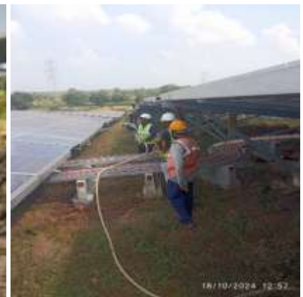
Solar Module Cleaning
