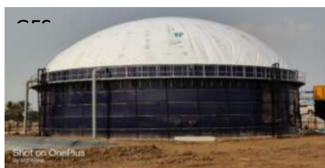
GFS Digester Tank (Completed)
