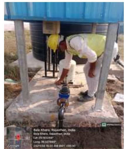
Testing of Pipeline with water
