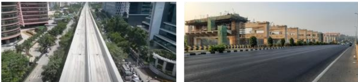
Figure 13: Metro construction progress on Outer Ring Road and Airport road
