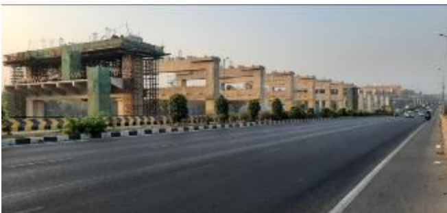
Images of construction progress
