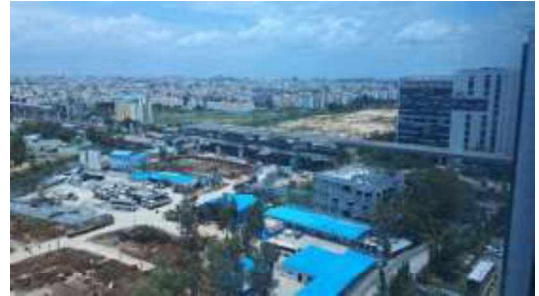
View of upcoming metro station close to Subject Project from upper floor of Subject Tower
