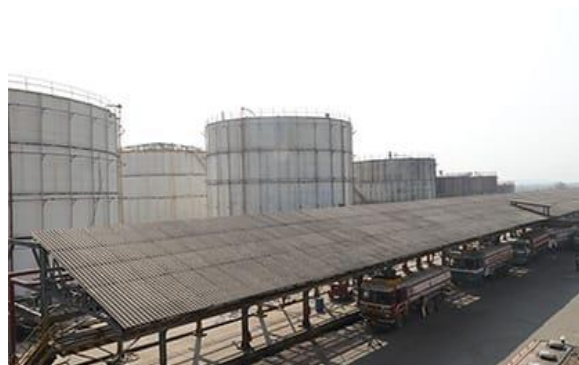
Storage for liquid products JNPT Terminal
