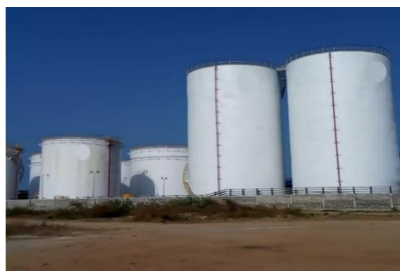
Storage for liquid products Deendayal Port, Kandla
