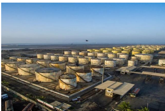
Storage for liquid products Deendayal Port, Kandla
