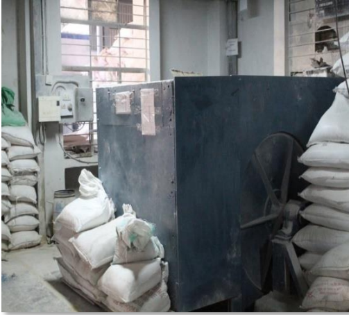
Ball mill-1- for crushing the raw material into fine powder
