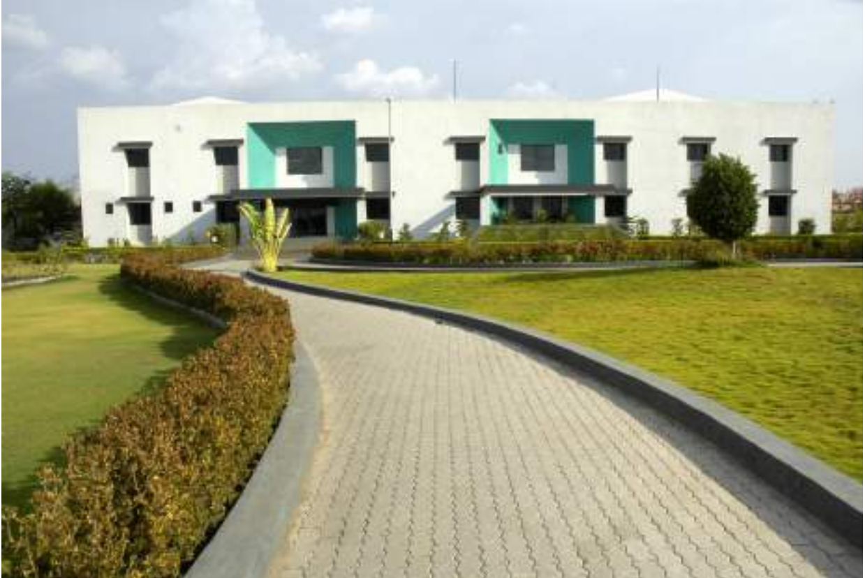
Machine Shop Building
