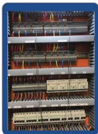
Power Distribution Industrial Panel
