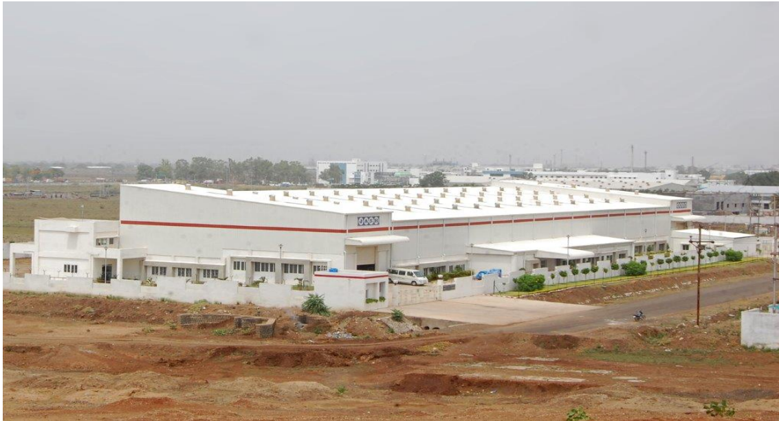
Exterior View - SEZ Export Plant III: Pithampur, Indore
