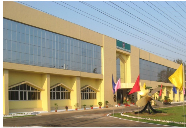
Steam System Repair Infrastructure at Naval Dockyard, Visakhapatnam
