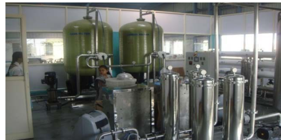
Reverse Osmosis Plant
