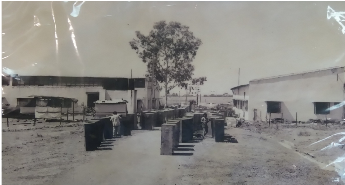
Decades back initial phase of above Manufacturing Facility as setup by Late Shiv Kumar Jhalani (Stock of Distribution Boxes)
